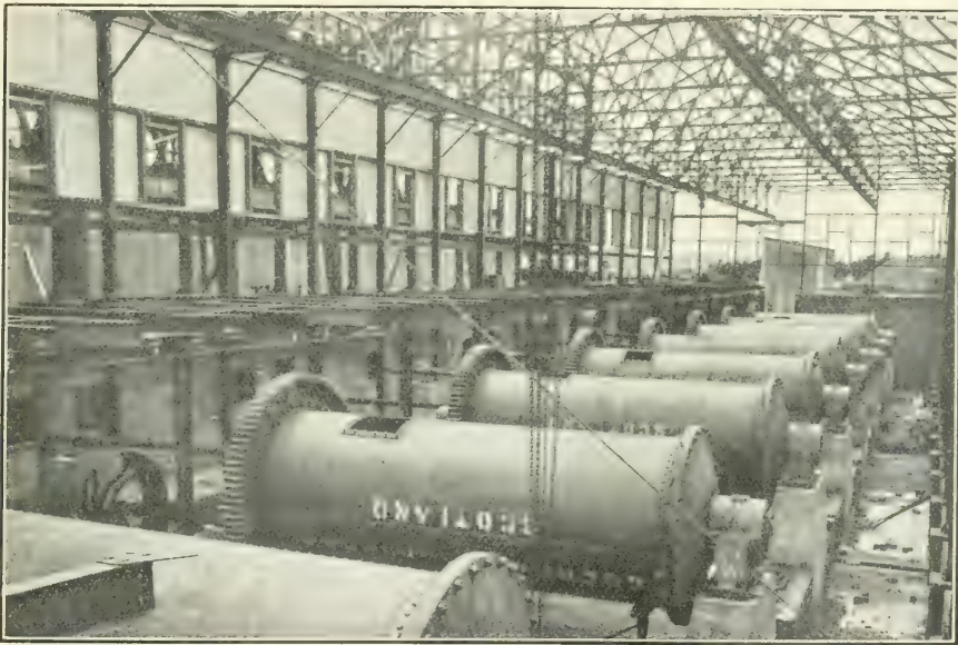
TUBE-MILLS AT VAN RYN DEEP, DURING COURSE OF ERECTION.
